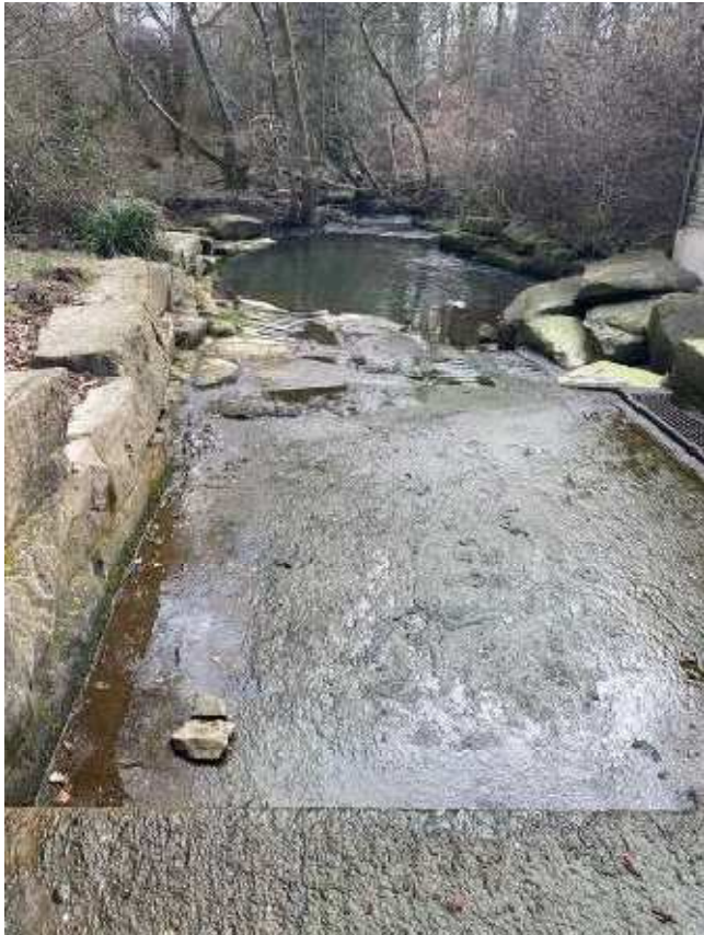
End of spillway
